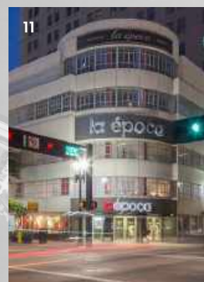
11 JULIA & HENRY'S FOODHALL Under construction for a 7 story multilevel entertainment complex that will include a rooftop restaurant, a basement speakeasy-themed bar, and three floors dedicated to more than 20 food and beverage concepts.
