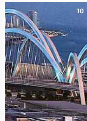
10 SIGNATURE BRIDGE Will carry a key segment of I-395 over NE 2nd Avenue and Biscayne Boulevard and redefine the Miami skyline with its six sweeping arches.
